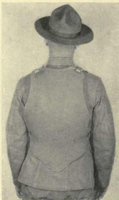
Fig. 199. Light body armor. Experimental backplate. American model, pressed in single piece
